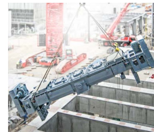
5. Double cooling screw conveyor
